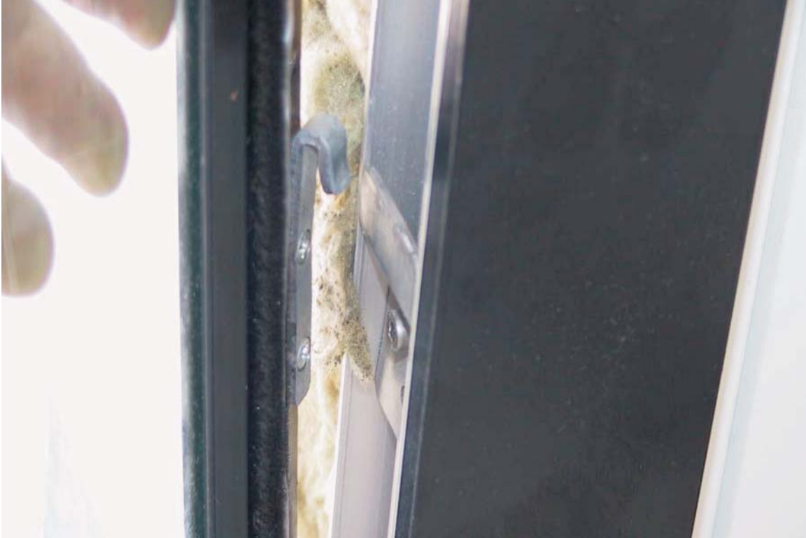
Glass panel installation.
