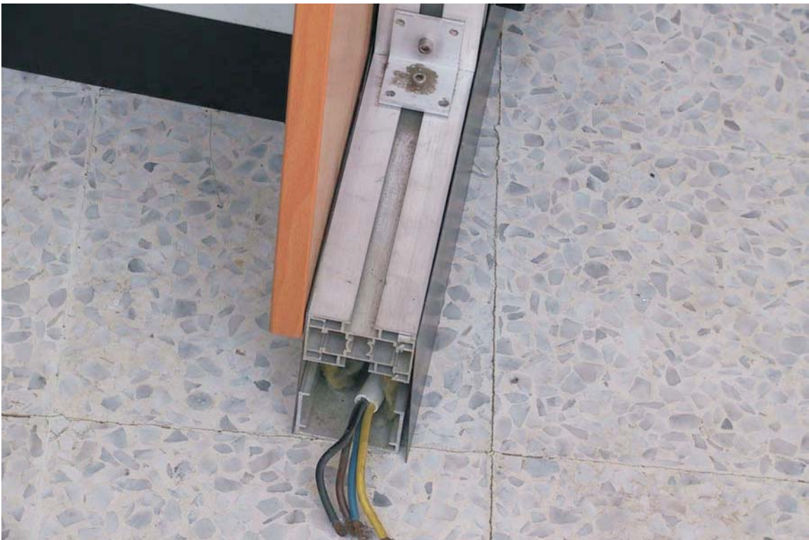
Skirting with Cable integration
