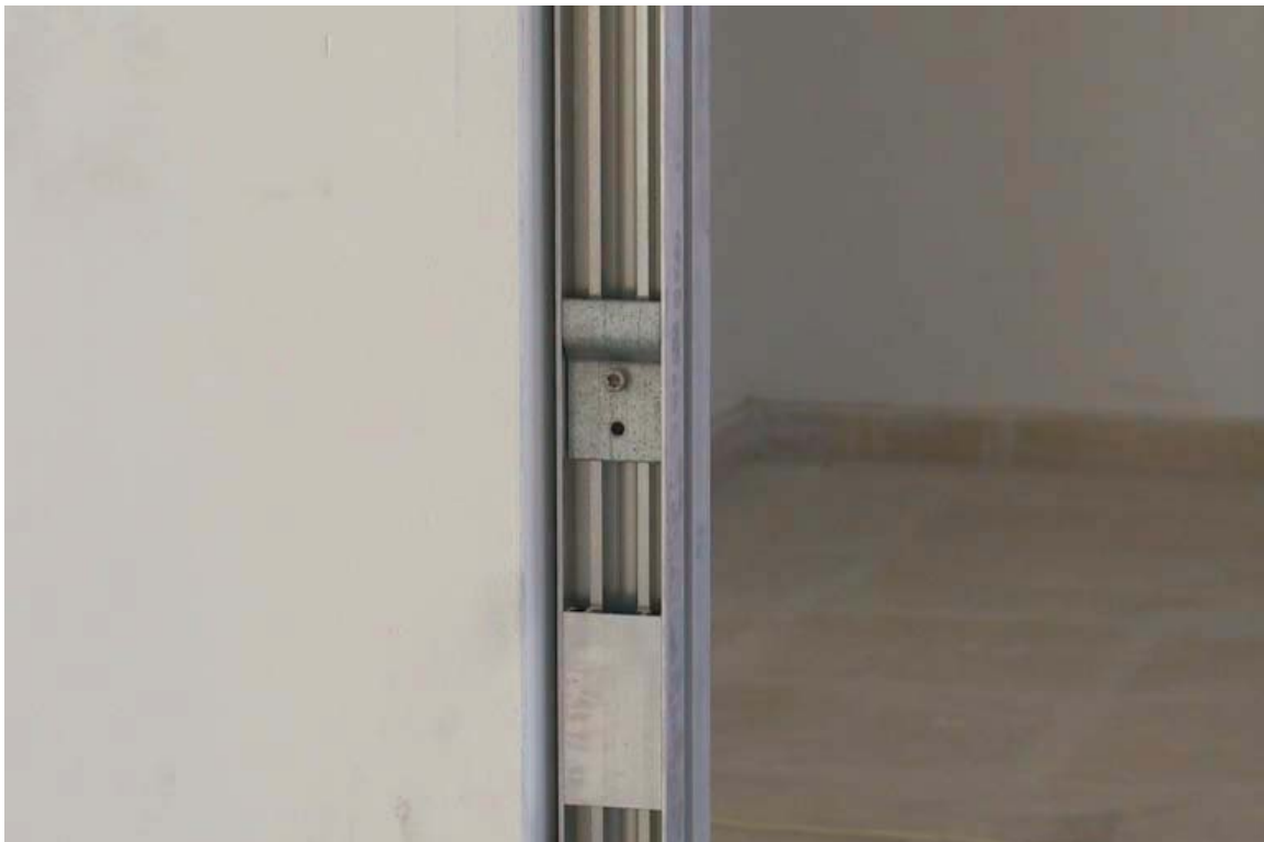
Main profile with hook stands and skirting clip
