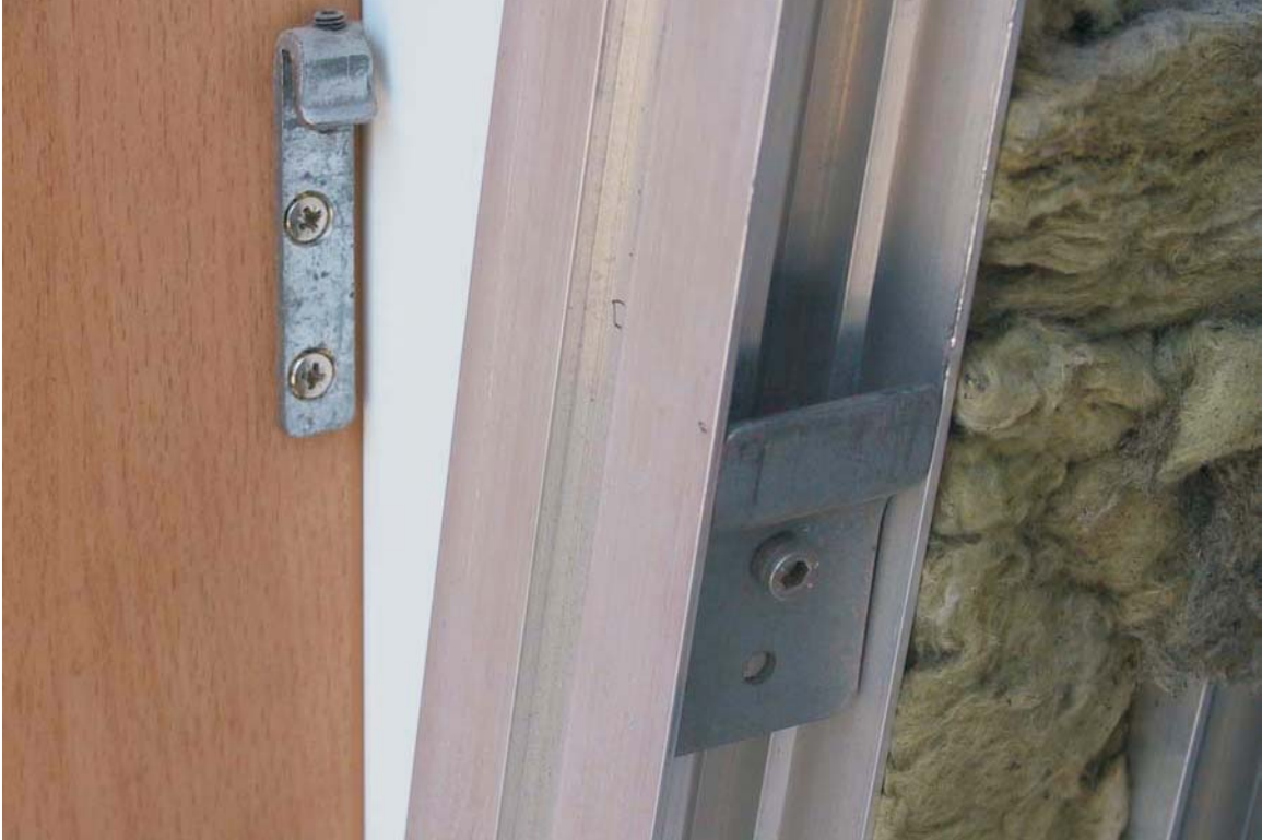
Wood Panel Installation
