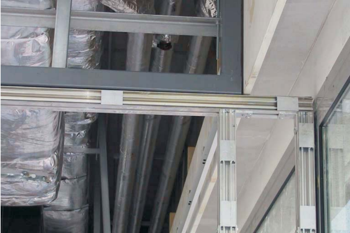
Metallic structure above F.C.
