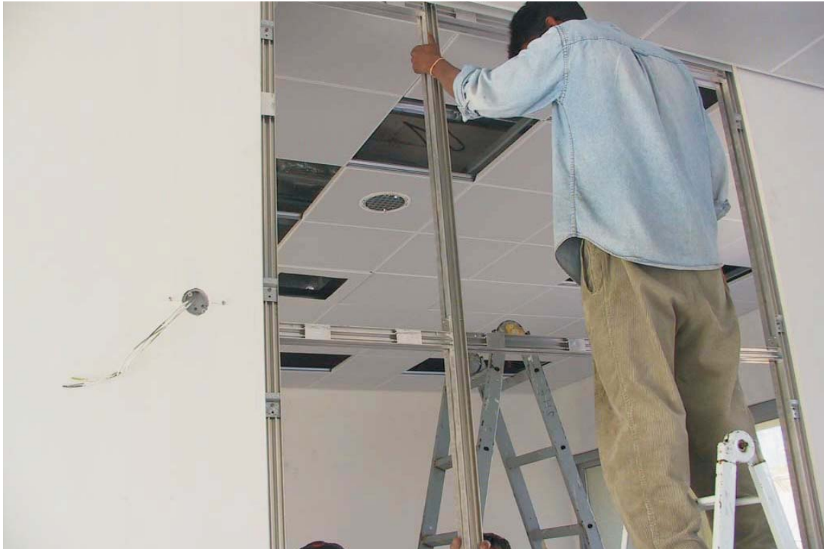
Structure with cover for inner skirting
