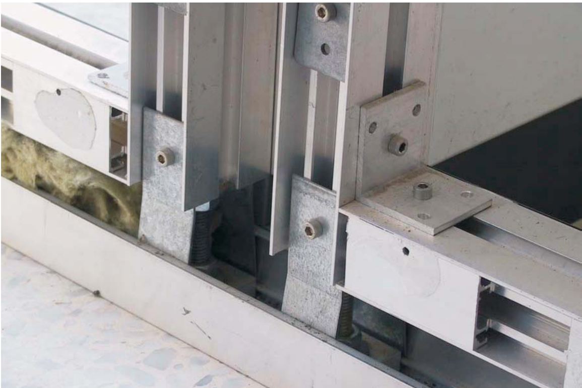
T Connection Lower detail
