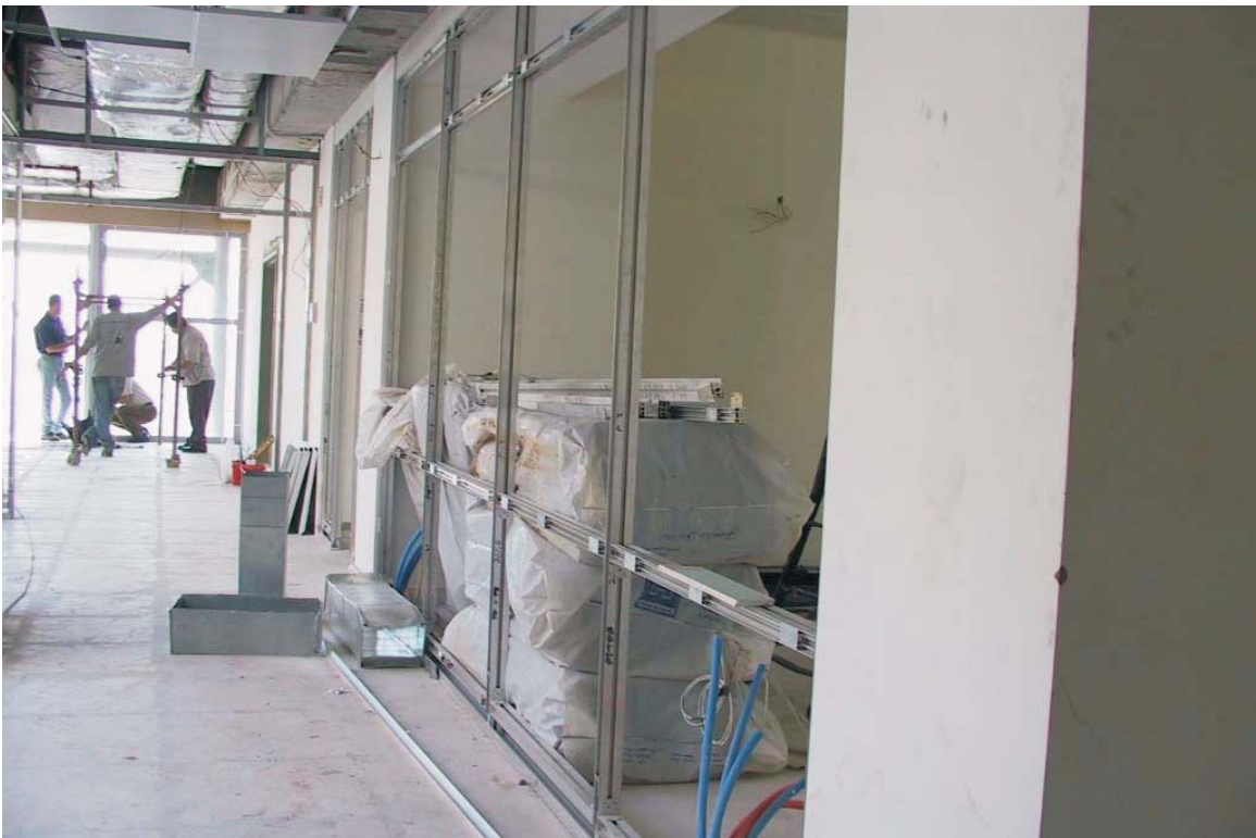
Wall structure with 3 levels
